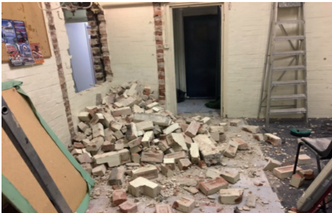
Creation of the through corridor between dressing rooms
